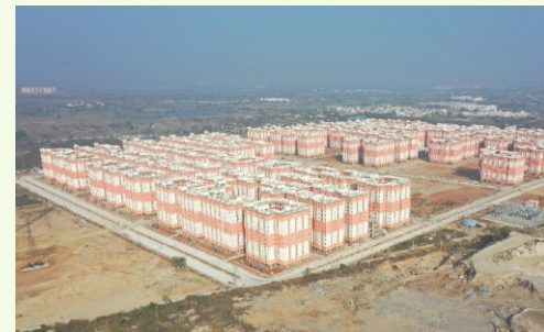
Site view of AHP-Kollur-Phase-II of GHMC
